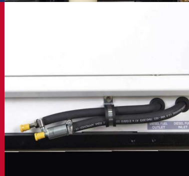
Input/output fuel pipe
