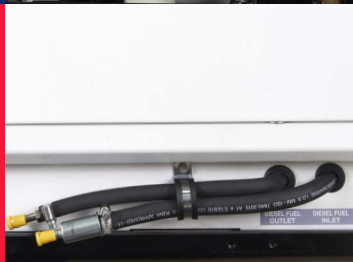
Input/Output fuel pipe
