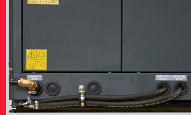
Input/Output fuel pipe
